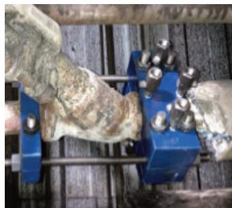
Weld Enclosure With Strongback
